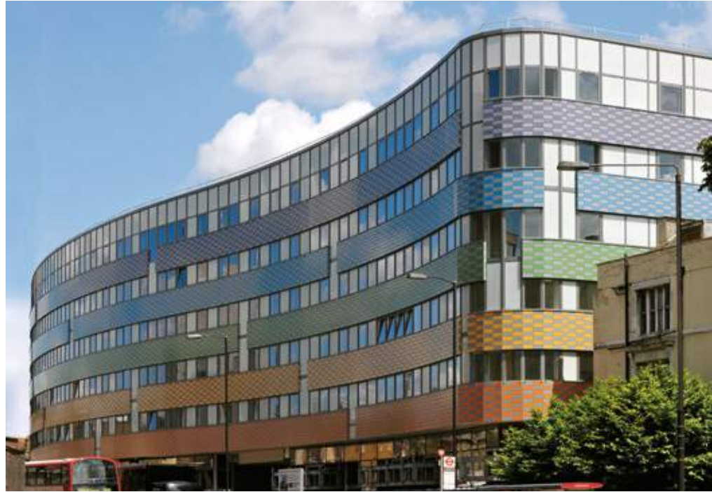
Students' hall of residence Isledon Road, London, Great Britain / Architect: TP Bennet
