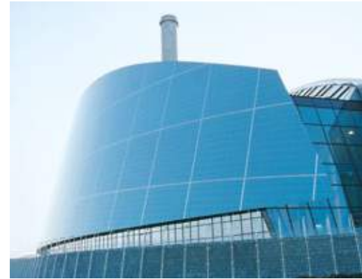
Thermal power station, Viborg, Denmark / Architect: Peter Kjelgaard & Thomas Pedersen M.A.A
