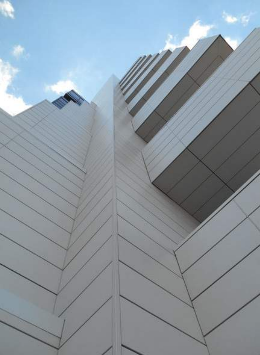
The new building shell
